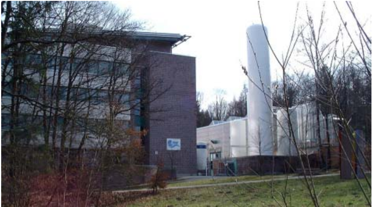
Fig. 11: ZSW Buildings and fuel infrastructure ( H_2 , O_2 , CO_2 , N_2 , CO , CH_3OH )
